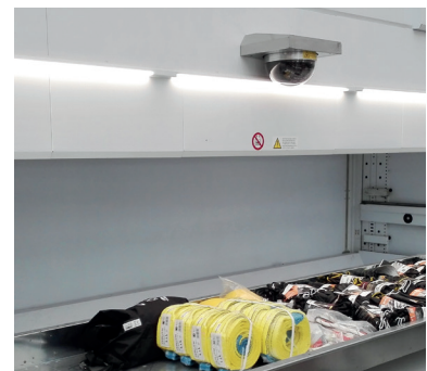
External bay lighting
