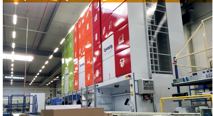
Fire protection system integration
